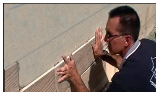
Work the tile onto the wall using a left-to-right motion.
