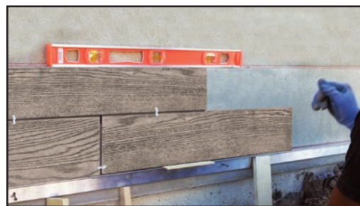
Use a rigid aluminum channel to support and level the first row of tiles during installation.
