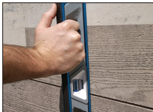
Use a large level to check and maintain an even-face plane over multiple tiles.
