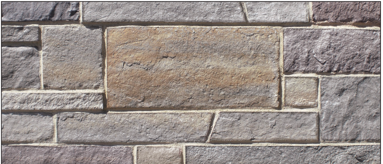
1/2" Deep Raked Grout Joint
