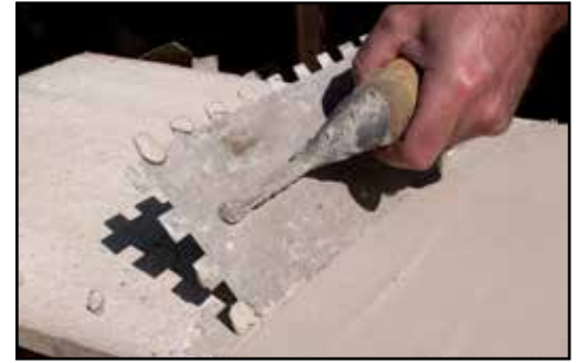
Apply a thin polymer-modified thinset bond coat to the back of the stone.
