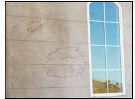
Mark all the low areas and use thinset to level them out to the proper height before installing Classic Series tiles.
