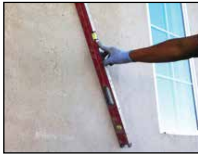
Use a long level or straight edge to confirm your wall is flat.
