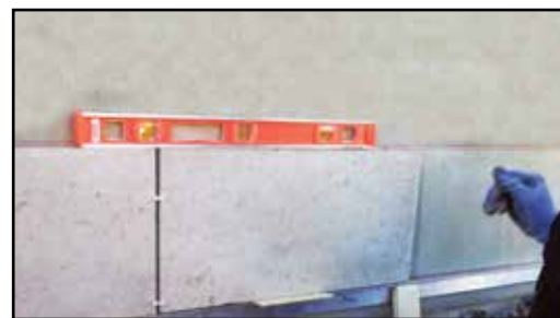
Using a propped up rigid aluminum channel can help you support and level out the first row of tiles during installation.
