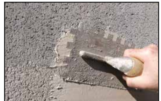
Apply a polymer-modified thinset bond coat to your substrate.
