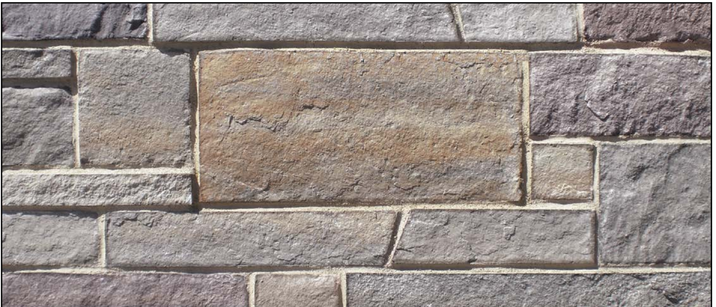
1/2" Deep Raked Grout Joint
