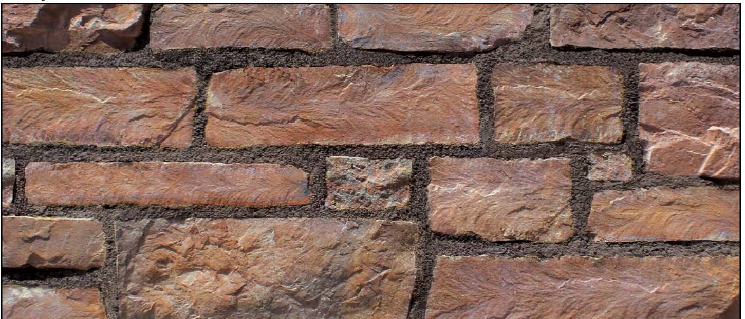
½" Deep Raked Grout Joint
