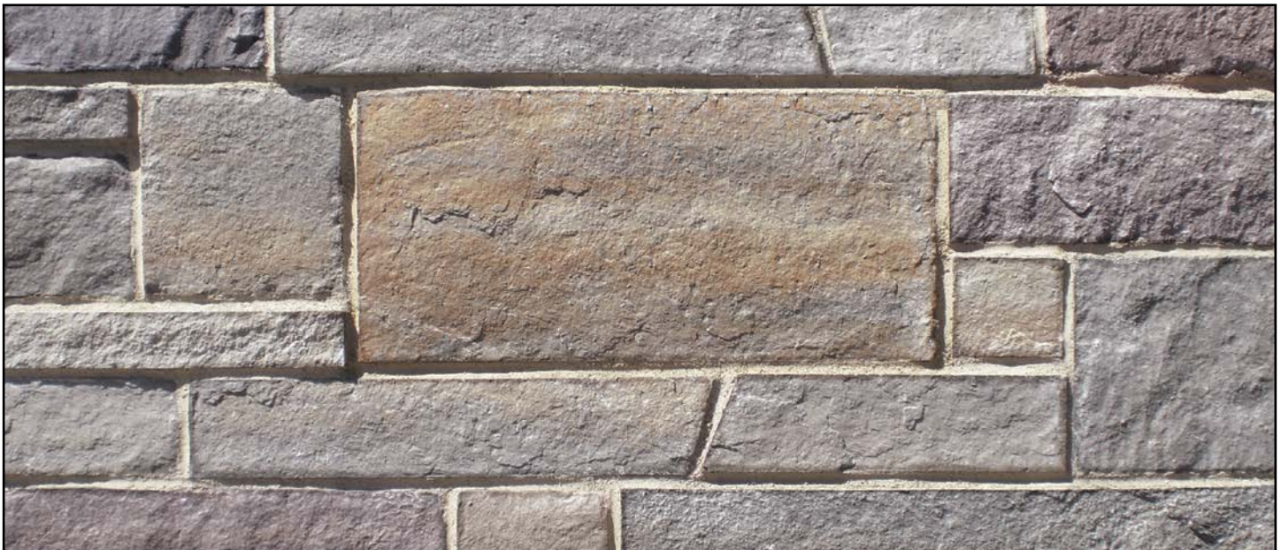
1/2" Deep Raked Grout Joint
