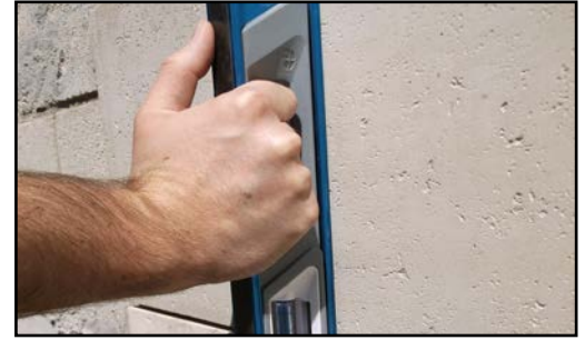
Use a large level to check and maintain an even-face plane over multiple tiles.
