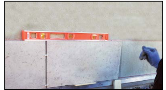
Using a propped up rigid aluminum channel can help you support and level out the first row of tiles during installation.
