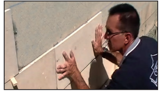
Work the tile onto the wall using a left-to-right motion.
