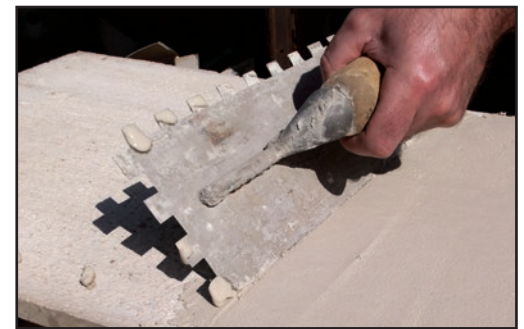
Apply a thin polymer-modified mortar bond coat to the back of the stone.
