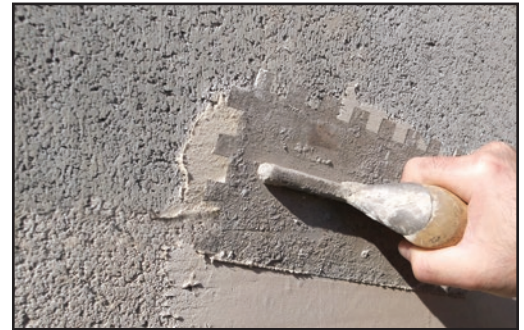
Apply a polymer-modified mortar bond coat to your substrate.
