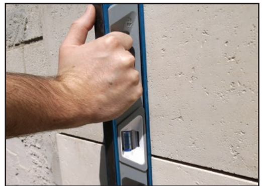
Use a large level to check and maintain an even-face plane over multiple tiles.
