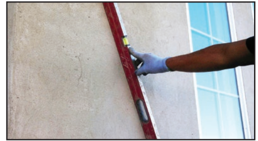
Use a long level or straight edge to confirm your wall is flat.
