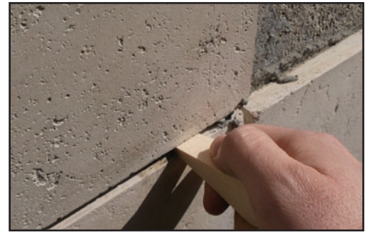
Spacers should be used to maintain uniform joints.
